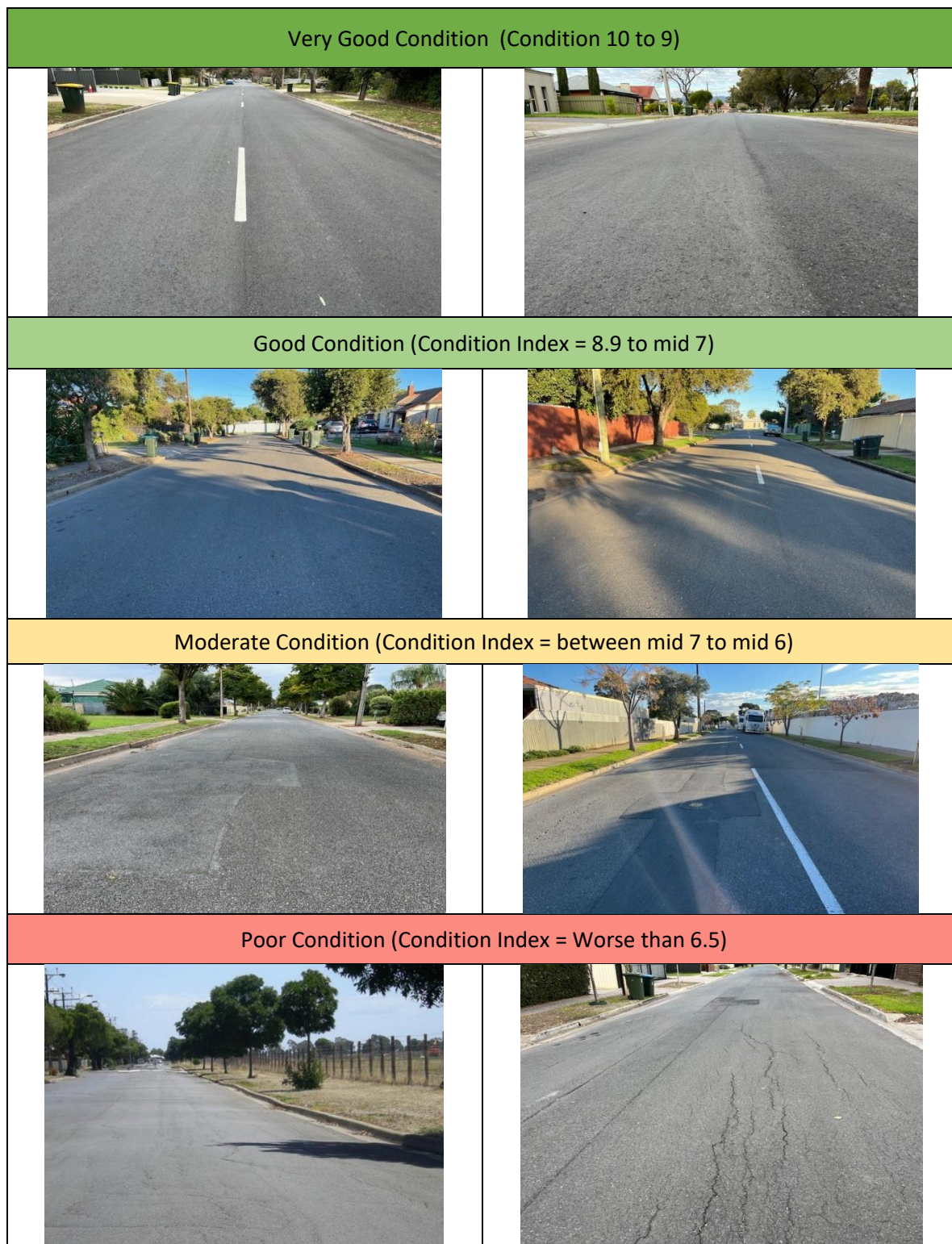
Image 6.2.1: How a road may present within our condition range
