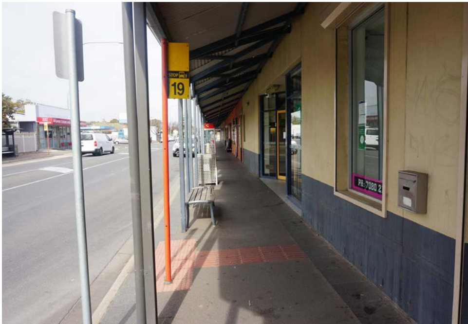
② Pedestrian walkways under the building canopy
