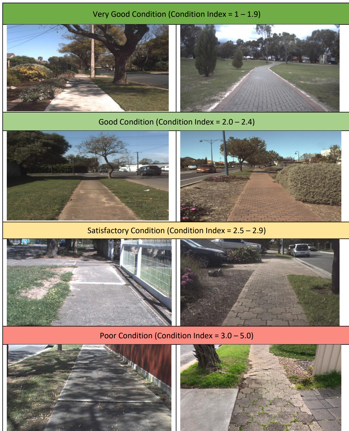
Image 6.1.1: Understanding our footpath condition range by photo
